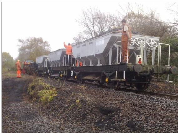
From the archives 2 : scenes from November 2009 :- The WRT 'Dogfish' wagons being put to use at the work location at Broken Banks in November
