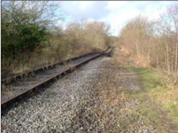
From the archives ; the scene at Broken Banks near Bishop Auckland in 2007 and now after the recent rain further remedial work will need to be carried out. (Photo : John Askwith)
