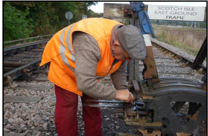
Roly Johnson carrying out final adjustments to the ground-frame locking at Scotch Isle East. See news item. (Photo : Trevor Horner)
