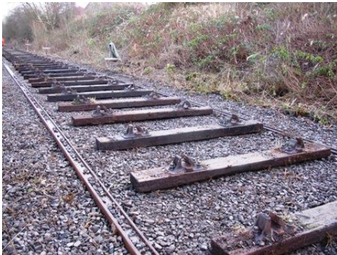
New track layout being prepared at Broken Banks
