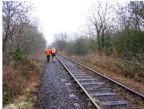
The line after reinstatement
