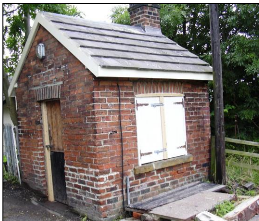
Witton le Wear Crossing Keepers Cabin, progress Photo, roof complete, window in place( T Hewitt)
