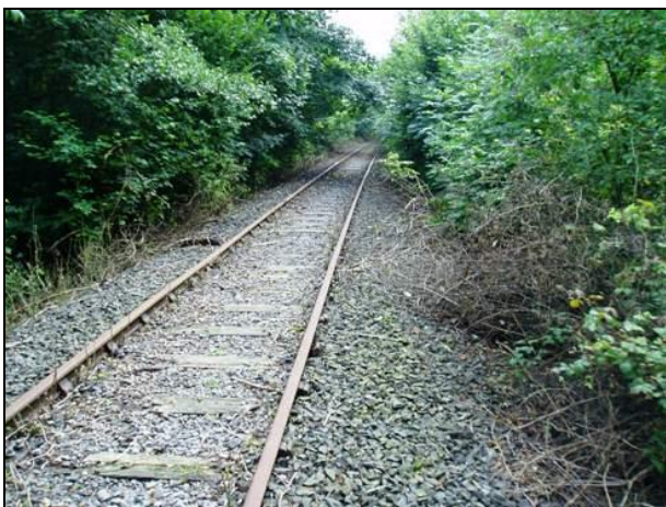
Two more before and after photographs of the permanent way between Wolsingham and Witton le Wear – showing the results of vegetation clearance, reballasting and resleepering.( A Gregory)
