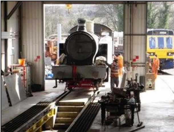
No 40 moved out of the Depot at last to have the cab roof replaced. Taken on 18 th March. (Photo : K McNally)
