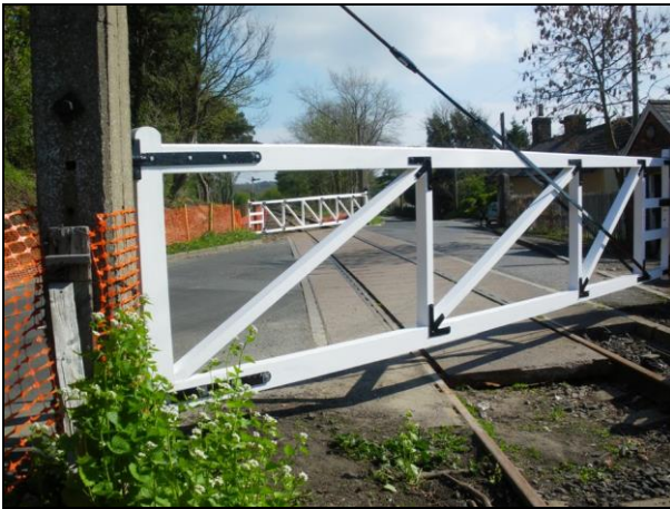
A view of the two gates newly installed at the Witton le Wear level crossing looking east. The nearest gate is 21ft in length , the far one 35ft. ( Photo : David Scott)
