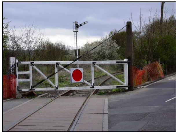
Looking west a couple of days later with the tensioning and mesh in place. Shouldn't that signal be at 'danger' now? (Photo : T Hewitt)
