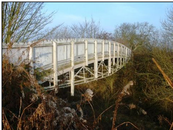
Bridge 12 near Escomb Village – a Grade 2 listed skew bow spring bridge before work began.( T Horner )
