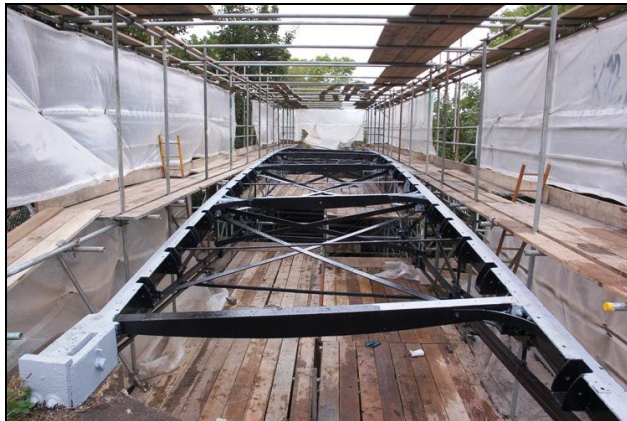
Bridge 12 with work underway on the wrought and cast iron members. (Photo T Horner)
