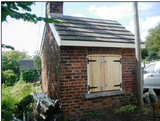
The Witton le Wear Crossing keepers cabin restoration continues – the east side windows and shutters in place (Photo : D Scott)
