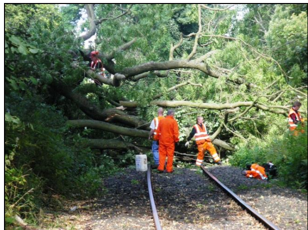
Parsons Byers : 1 September – fallen trees block the line RMS & WR staff and volunteers start the clearance work. ( Photo : D Scott)
