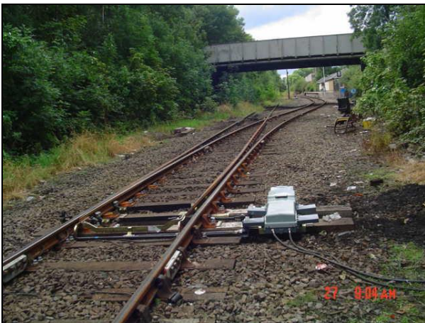
Bishop Auckland, looking west: The completed turnout with new point motor, Weardale line runs straight ahead (Photo M Westerfield)
