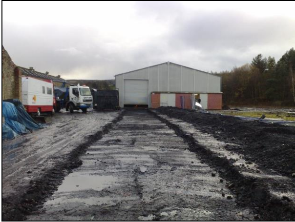
A view looking towards the main shed with the ground prepared for the new siding extension –leading from the rear of the main depot shed) The effects of the recent spell of wet weather are evident. (Photo : A Gregory )
