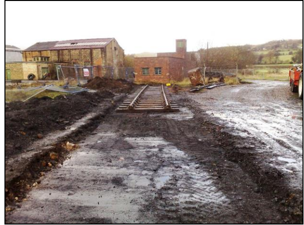
Looking in the opposite direction (towards the road) with the first section of track in place. The red brick building will be demolished to allow the loading siding to be extended. ( Photo : A Gregory)
