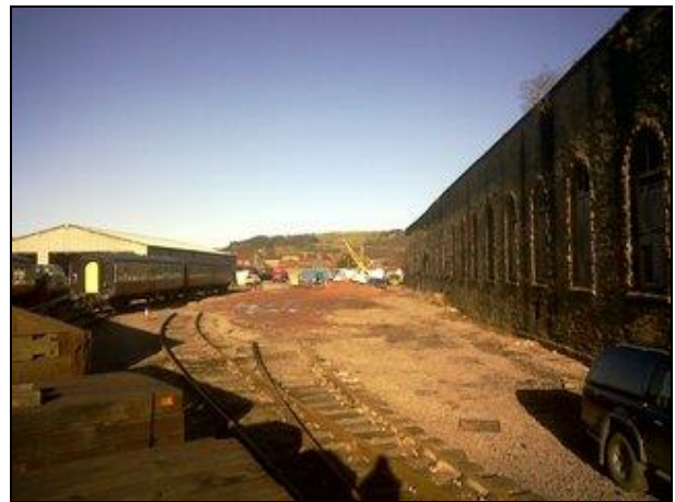
The former sidings yard at Wolsingham now cleared in preparation for the laying of the main siding and the coal loading area. See map in last issue. ( Photo : A Gregory )
