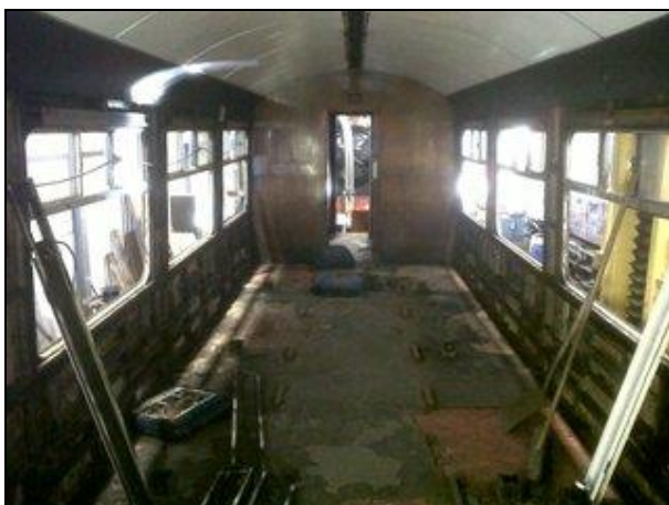
WRJC Coach with seats, tables, toilets and ,luggage racks removed. Internal walls and floor panels will be replaced
