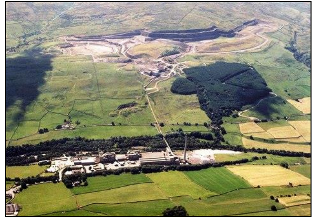
The Eastgate site looking south over the works and on to the quarries on the slopes beyond. The works site is now cleared.
