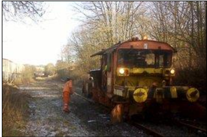
The Ballast Regulator at Bishop Auckland, job done. (Both photos A Gregory )
