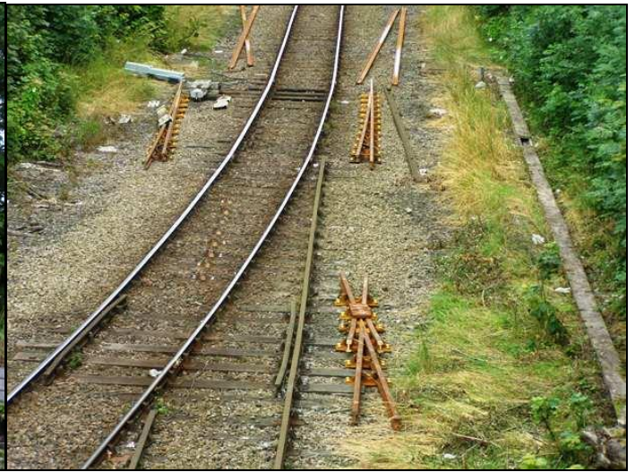
Bishop Auckland station east end looking towards Darlington with new point-work on site ( Photo :K Hillary)
