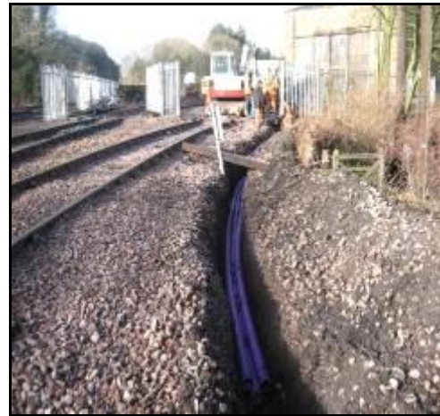
Ducting for cables being prepared outside the Depot (Both photos : N Swindle)
