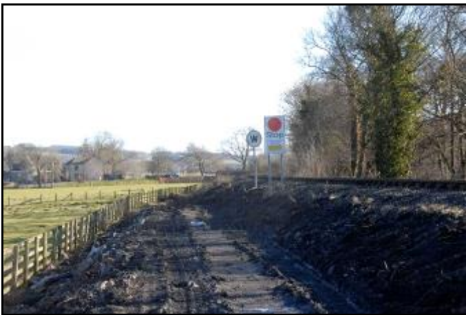
These two photos indicate the considerable volume of fill required to make the loop line up to the grade level of the main line. On the left looking east at Scotch Isle and on the right looking back towards the Depot at Wolsingham. (Both Photos : J Lewins)
