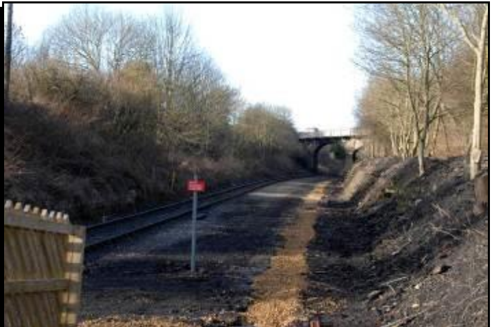
A siding is to be laid at Bishop Auckland to allow a train to or from the Network to pass a WR passenger train standing at the platform. On the left is the trackwork and sleepers for the turnout laid out at the depot (Photo N Swindle) and on the right the trackbed preparations looking from the platform towards Latherbrush Bridge. (Photo : J Lewins)
