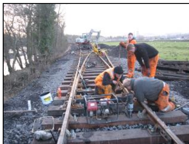
Two views of the west end of the loop with turnout installed. This work was carried out by the BARS track construction Company – RMS Locotec under the direction of Alistair Gregory and Steve Goodwin. They both send their thanks to all involved ( Photo left : S Goodwin and right : N Swindle)
