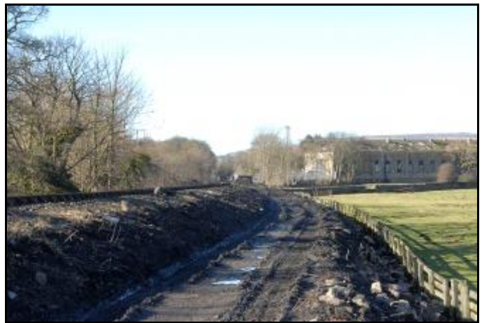
These two photos indicate the considerable volume of fill required to make the loop line up to the grade level of the main line. On the left looking east at Scotch Isle and on the right looking back towards the Depot at Wolsingham. (Both Photos : J Lewins)
