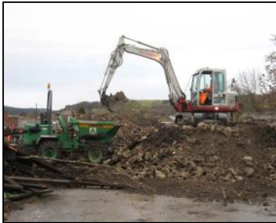
Some of the fill required for the new line came from demolished buildings in the Depot (above) also from the site of the former Down platform at Wolsingham.
