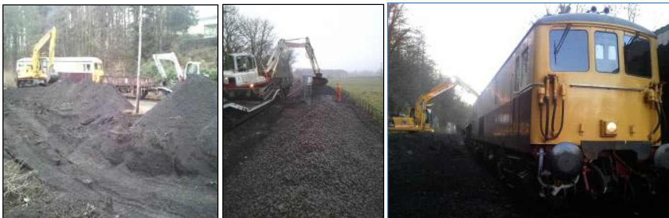
More progress photos : excavating the fill , loading onto a Class 73 hauled works train and unloading the fill at the worksite. (All photos : A Gregory )
