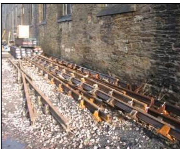
A siding is to be laid at Bishop Auckland to allow a train to or from the Network to pass a WR passenger train standing at the platform. On the left is the trackwork and sleepers for the turnout laid out at the depot (Photo N Swindle) and on the right the trackbed preparations looking from the platform towards Latherbrush Bridge. (Photo : J Lewins)
