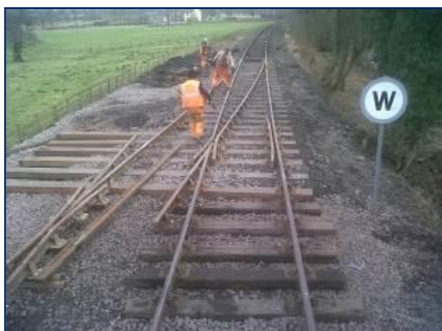
Two views of the west end of the loop with turnout installed. This work was carried out by the BARS track construction Company – RMS Locotec under the direction of Alistair Gregory and Steve Goodwin. They both send their thanks to all involved ( Photo left : S Goodwin and right : N Swindle)
