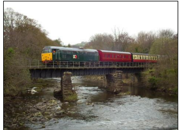
31601 heads the morning train across Broadwood bridge on the first day of the 2012 season, April 6. Photo : Chris Simpson.
