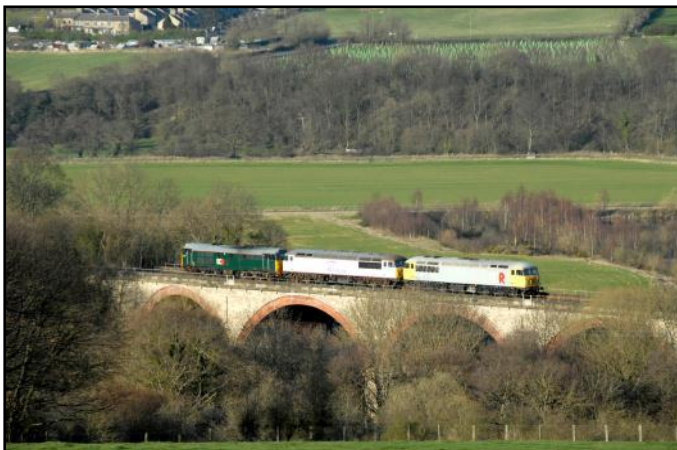
31601, 56091 and 56311 cross Etherley viaduct on 27 March near the end of its journey from Washwood Heath (near Birmingham) to Wolsingham. Photo : John Lewins.
