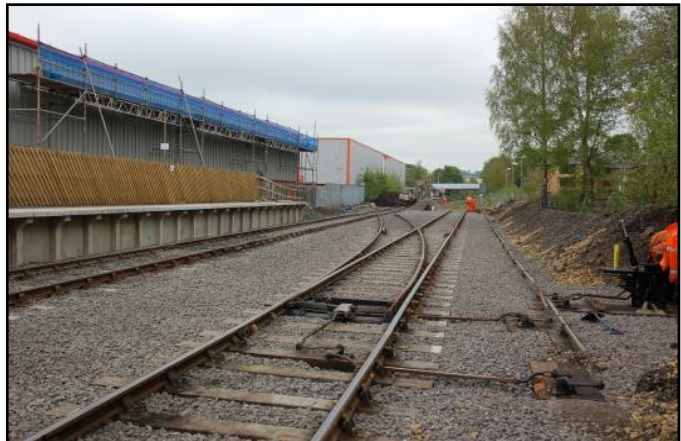
The completed work on the east end of the Bishop Auckland loop with the ground frame and ballasting completed. (Photo : Trevor Horner)
