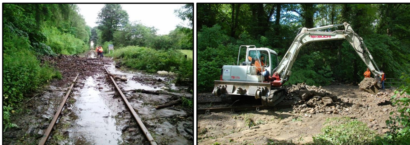
Just to the west of Bridge 18, a culvert overflowed onto the line carrying yet more rock onto the line , RMS moved in under the direction of Civil Engineer Brian Green and removed the debris the next day in preparation for the following days train services. Photos : Alistair Gregory.
