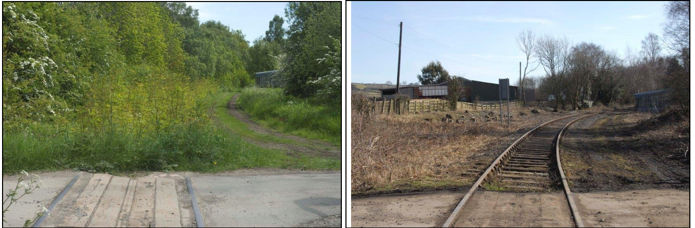
Enginemans Terrace , looking towards Wear Valley Junction. Two views: on the left taken in 2008 and on the right, the same view taken in mid March 2010 after clearance work by the Sunday gang and the team from RMS. The hut on the right provides a reference point. ( Both Photos : J Lewins )
