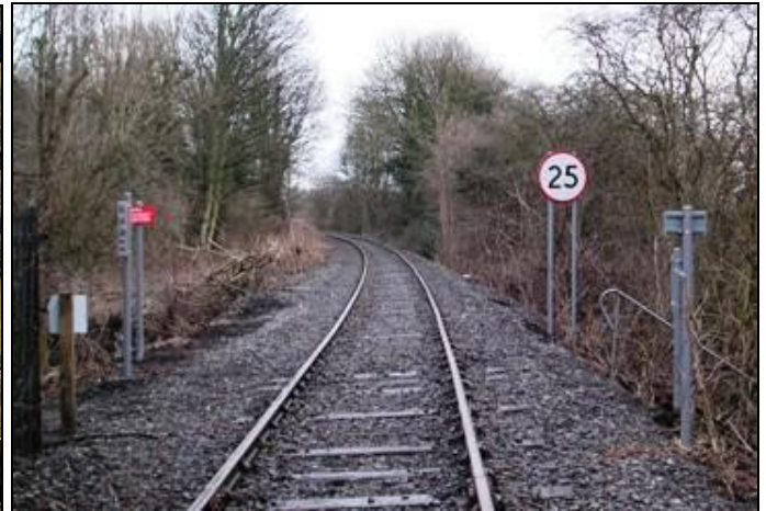
Footpath crossing near Witton le Wear after the erection of signs - there are six required in this case . (Photo : S Bissell)
