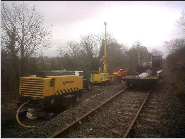
Broken Banks : Borehole drilling to examine the subsurface Geology (Photo : A Gregory )
