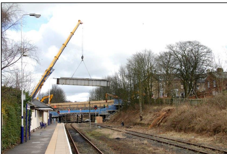
COCKTON BRIDGE at Bishop Auckland is now being replaced, necessitating both traffic diversions and train service substitution. On the left a photo from J Lewins showing the last section of the old bridge being lifted clear ( April 3 rd ) and on the right one of the deck sections being lowered in the parking area at the rear of the station – photo : K Hillary.
