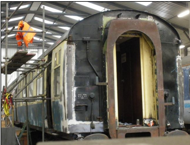
Recently completed welding on the coach ends of ‘Nina’ in the Depot at Wolsingham . (Photo : D Scott)
