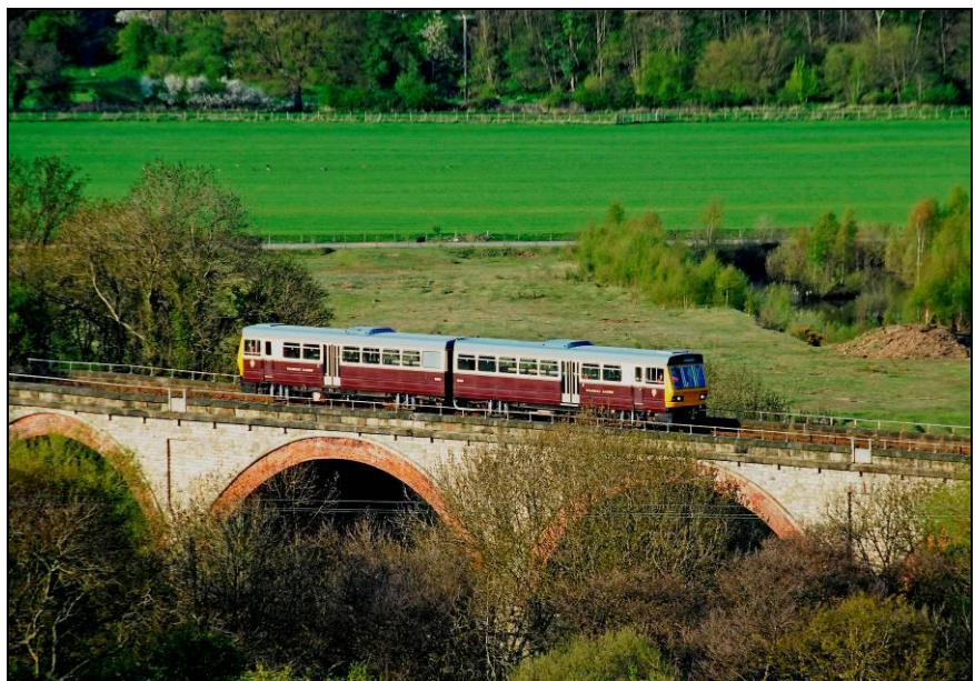
Heading for Bishop Auckland , the 141 which will be the mainstay of the Community service crossing Etherley Viaduct on a crew training trip on 4 May (Photo : J Lewins)
