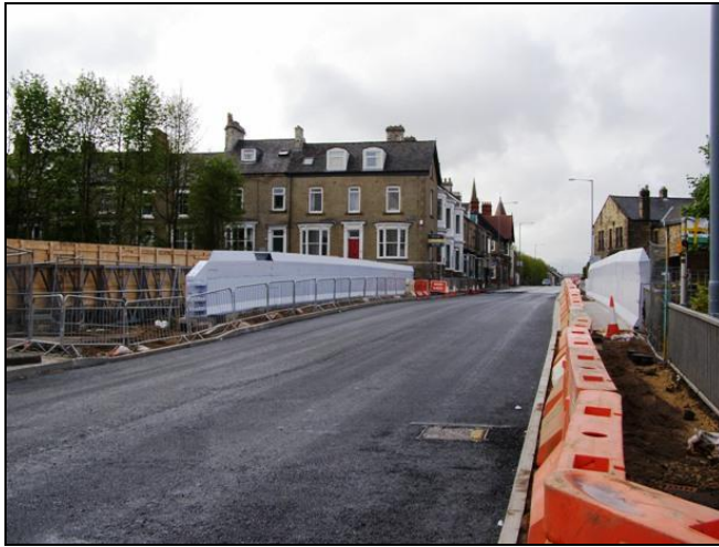
Cockton Hill bridge – May 12 – the work on the new bridge nearing completion. (Photo : K Hillary)
