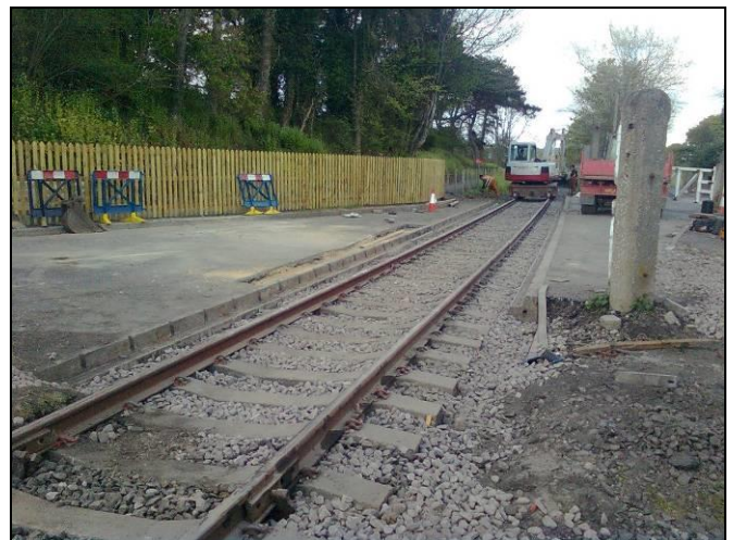
Witton le Wear level crossing with track restored and ready to replace road panels- taken on May 15 th . ( Photo : S Goodwin)
