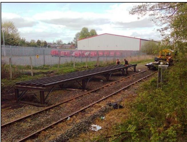
Work starts on the prefabricated platform at Bishop Auckland - taken on May 15 th ( Photo : S Goodwin)
