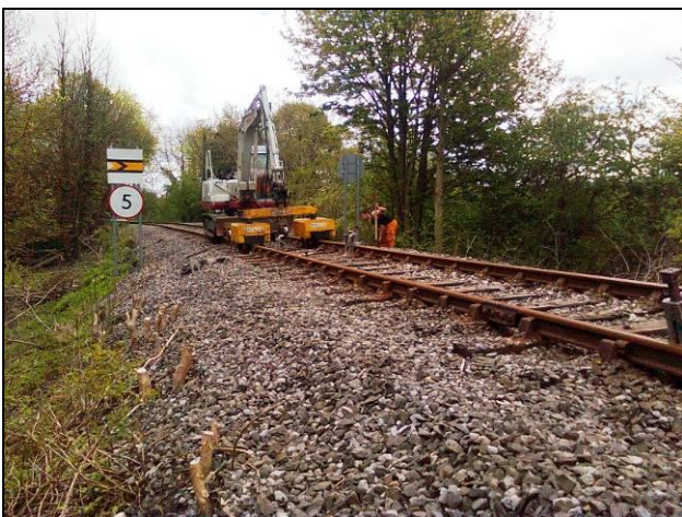
Project Connect : Road-Rail 360 with packing head, working on the ballast near Clemmy Bank. (Photo : S Goodwin)
