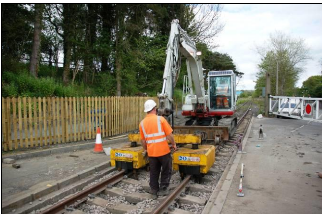
Jeff Smith directs Brian Mills with the tamping machine at the Witton le Wear crossing ( Photo : T Horner )
