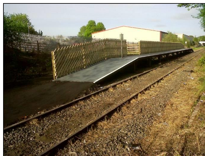
How to build a station platform in four and a half days. Top left : timber sheets laid on the prefabricated framework of used lengths of rail. Top right : painting of the platform surface , fencing in place. Bottom right, work underway on the fencing before the path down to the platform was surfaced and bottom right, the completed 40 m platform, which lies 150 m west of the Network Rail platform at Bishop Auckland. Photos : S Goodwin, except bottom left : A Gregory.
