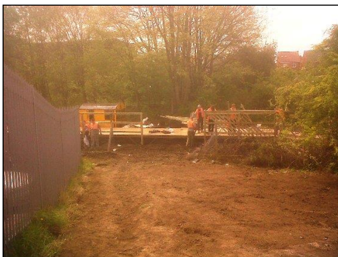
How to build a station platform in four and a half days. Top left : timber sheets laid on the prefabricated framework of used lengths of rail. Top right : painting of the platform surface , fencing in place. Bottom right, work underway on the fencing before the path down to the platform was surfaced and bottom right, the completed 40 m platform, which lies 150 m west of the Network Rail platform at Bishop Auckland. Photos : S Goodwin, except bottom left : A Gregory.
