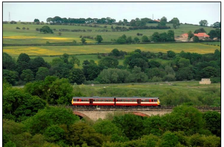
The second 141 class DMU( 141113)on service duty on the 20 th June seen crossing Etherley Viaduct ( Both Photos : John Lewins)
