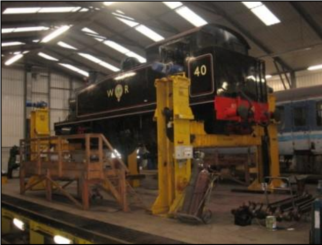
No 40 in the Wolsingham Depot raised on the jacks While undergoing work on the axles and bearings,
