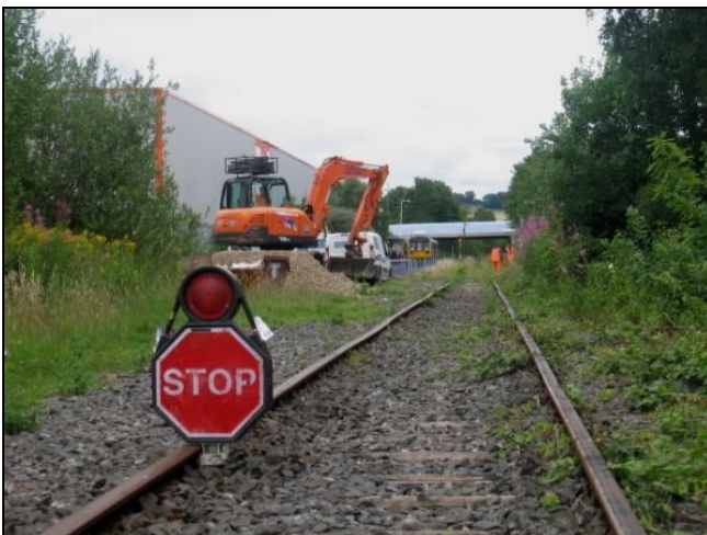
Drainage works underway on the land between the two platforms – this is where the planned linking path could be placed.
