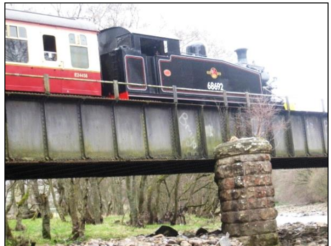
No 40 on Bridge 34 during the filming session for the ‘George Gently’ programme. It was converted to British Railways 69692 for the day. ( Photo : Norman Swindle)
