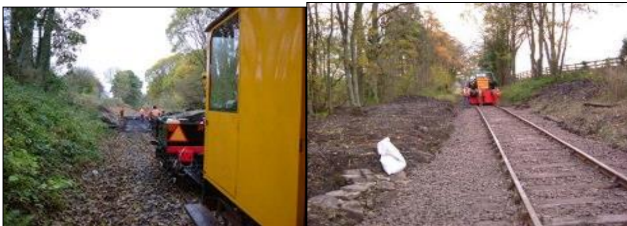
Parson Byers from the east showing work underway to rebuild the track profile View from the west with the track restored and re-ballasted
