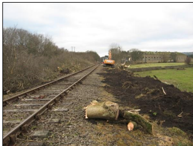
Two views of the work in progress extending the headshunt between Wolsingham Depot and Scorch Isle. On the left looking eastwards showing a stretch of the new track in position and on the right a view looking west towards the Depot showing the earthworks in situ for the next stage of the extension. (Both photos : Norman Swindle)
