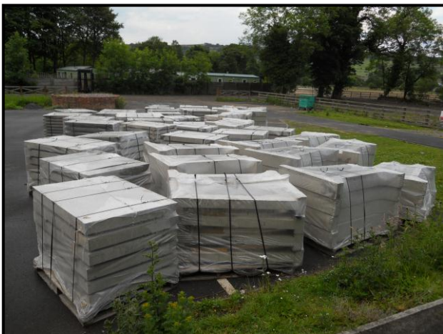
A view of the concrete sections for the new platform at Bishop Auckland West in the Wolsingham station ‘yard’. Photo : David Million
