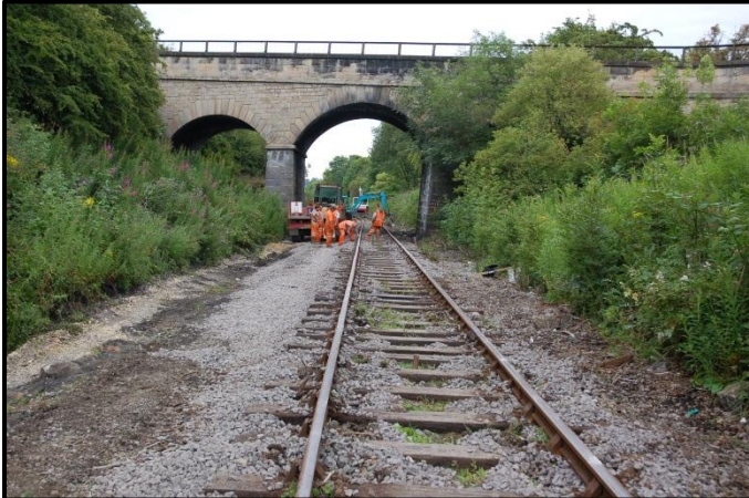
Bishop Auckland – Latherbrush Bridge. On the left a view looking towards the station with the RMS gang engaged in slewing the track under the bridge to provide room to install the turnout to the new siding. On the right a view in the opposite direction showing the area for the turnout. Both Photos : July 10 by Trevor Horner)
