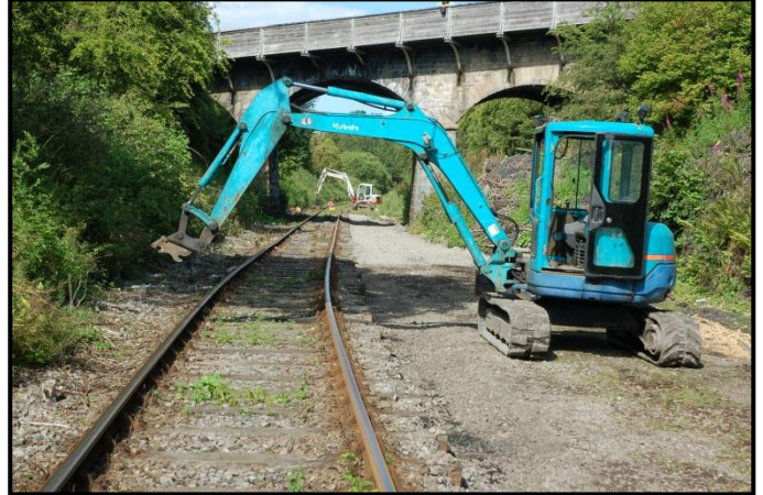
Bishop Auckland – Latherbrush Bridge. On the left a view looking towards the station with the RMS gang engaged in slewing the track under the bridge to provide room to install the turnout to the new siding. On the right a view in the opposite direction showing the area for the turnout. Both Photos : July 10 by Trevor Horner)
