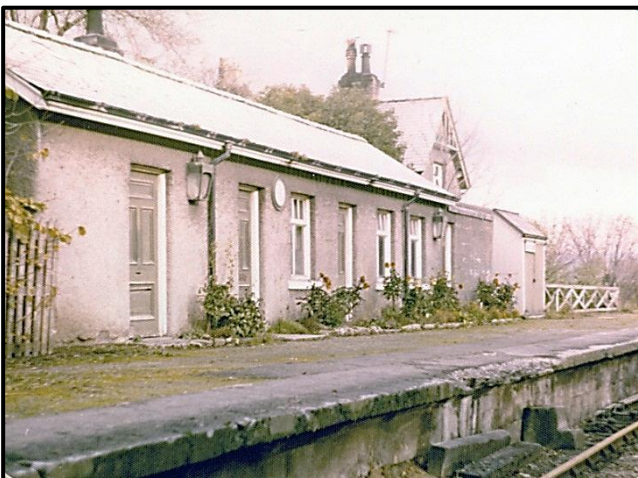
Taken in 1977 and already closed to passengers for 24 years this view shows that Eastgate station still had lamps, clock and signal frame box.
