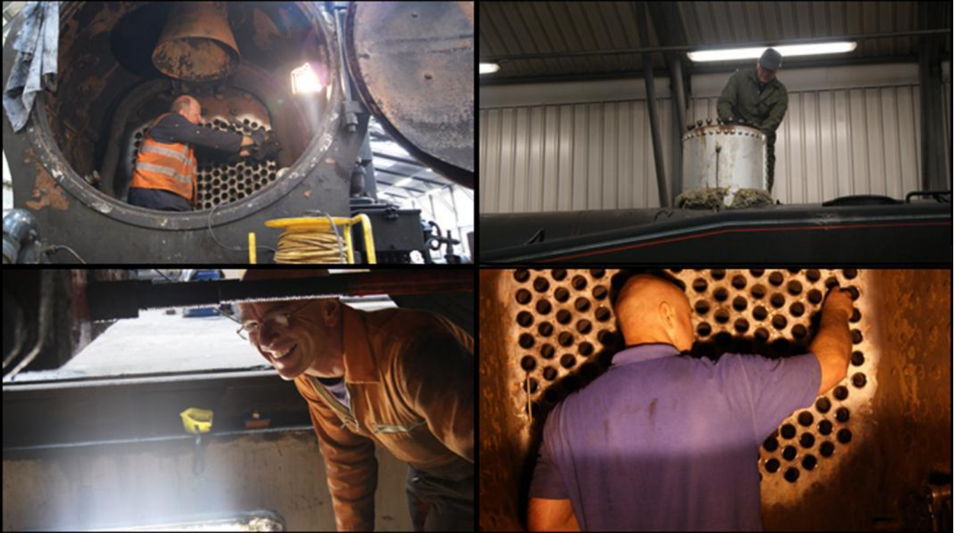
No 40 : Work continues on the Trust’s stream loco –here is a montage of progress photos taken by Ruth Carroll. As we go to press and after a satisfactory hydraulic test , the tubes are installed and expanded, the grate is in place and the brick arch is now being completed. The full steam test is planned for Thursday 26 th May and if all is OK No 40 will be back in operation on Sunday the 29 th .May.
