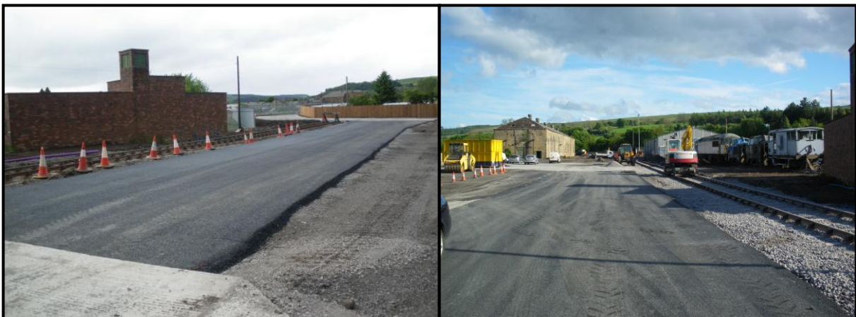
Work is progressing on the roadway into the depot, the turning circle for the lorries and, in the distance in the right hand photo the loading pad area. May 18 th . ( Photos : D Scott)
